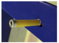
STEP 2: Please insert the four cap head screws with the yellow sleeve into these rivnuts. This will allow for the wall linings to be installed but keeping the threads clean and provision to install the face plate screws during the second fix. NOTE: These cap head screw will be discarded after the second fix.
