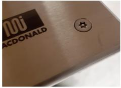
STEP 6:Once the push plate is aligned you should see the M4 rivnuts, fit the M4 security screws to secure the plate.
