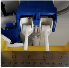
STEP 4:Using a straight edge, mark and cut the two push rods so that the cute edge is flush with the wall lining.
