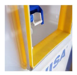
STEP 3: Follow the Wisa instructions and cut the yellow box section flush with the face wall. Then attach the two push rods to the tripper mechanism.
